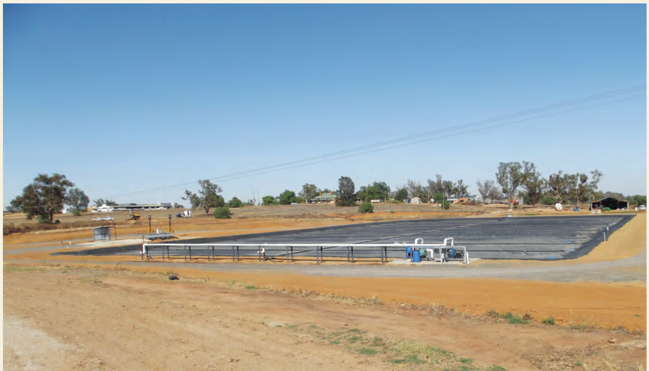
Rivalea’s biogas facility at Corowa captures and burns methane from effluent to reduce greenhouse gas emissions.
