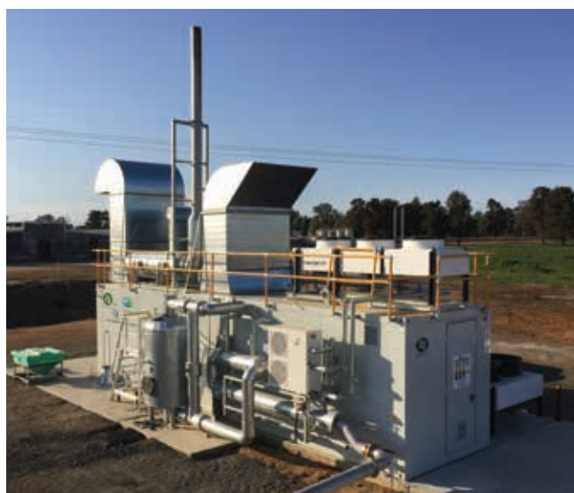
Rivalea's biogas generator with capacity to supply 25% of the Corowa site's power requirements
